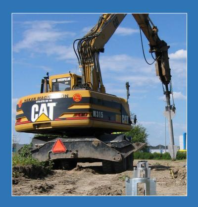
...Tracked machine with hydralic hammer or alternatively alternative excavator with hydraulic hammer used for knocking down
